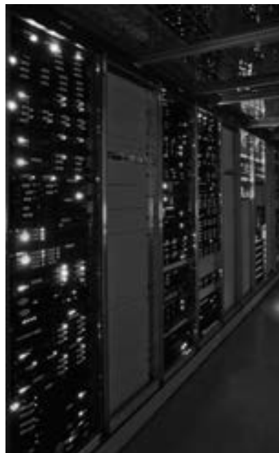
Blick ins Datacenter.
